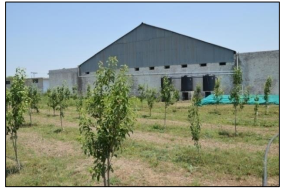
Rooftop rainwater harvesting structure to harvest rainwater
